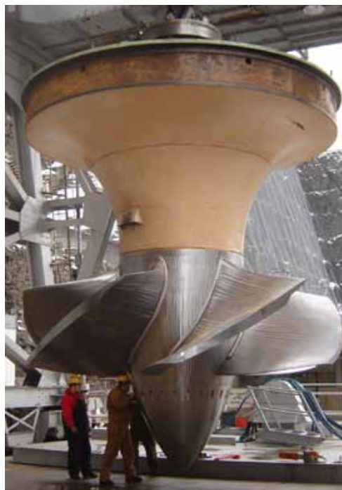
Noxon Rapids turbine upgrade
