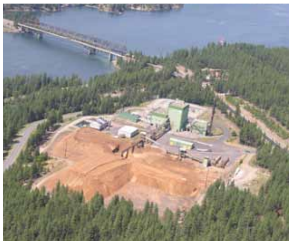
Kettle Falls Generation Station
