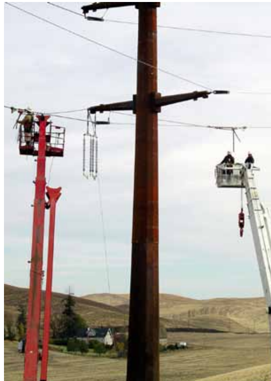
Transmission upgrade work
